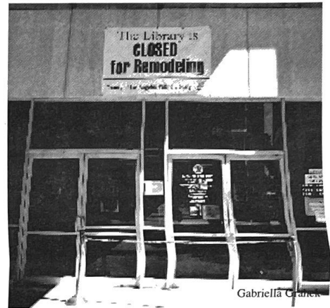
RENOVATION BEGINS: Construction begins at Malibu Library and the surrounding area
